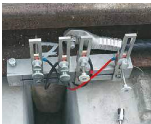
On site testing
