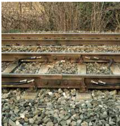
Transmission of coded and return current on lines fitted with automatic block
