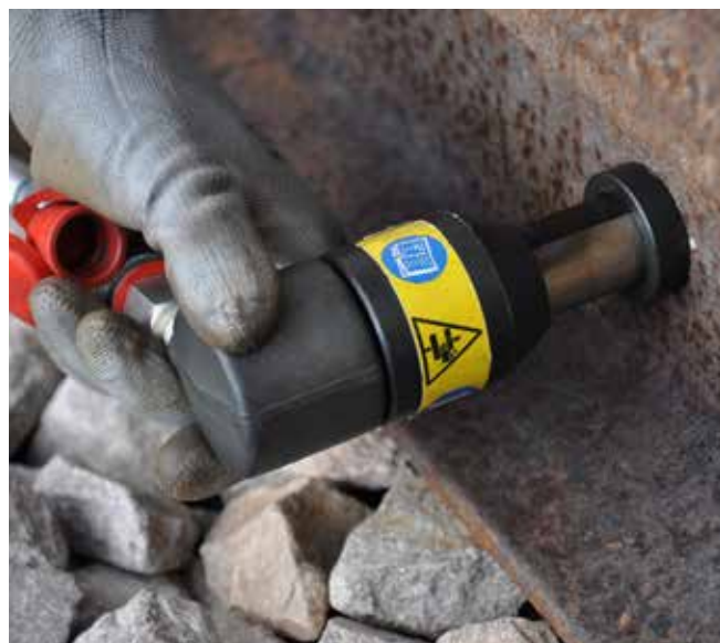
RHTEP while extruding AR contact
